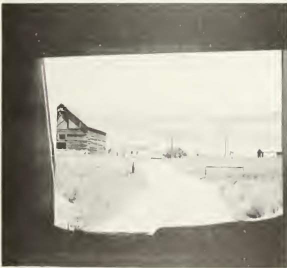
Looking North from NORTH ENTRANCE
